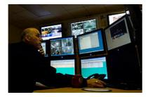
**The site survey** revealed a mixture of good electronic security equipment but a poor design in the way it was installed. The on site guarding located in the top of site control room could receive alarms if activity was detected on site. These alarms were not logged so a missed alarm, or disabled alarm was a common occurrence.
